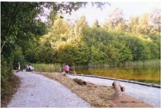
This is the most frequented fishing area. It once was slippery and very muddy. The Project workers have used all natural materials to shore up the bank. You can see the straw along the trail and sandbags piled along the lake edge. On Oct 1 we need to plant some shrubs and trees. Here are details of the logs, burlap and sandbags.
